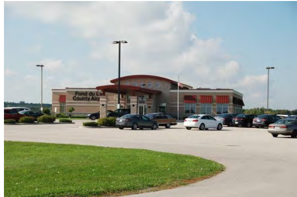
Fond du Lac County Airport
